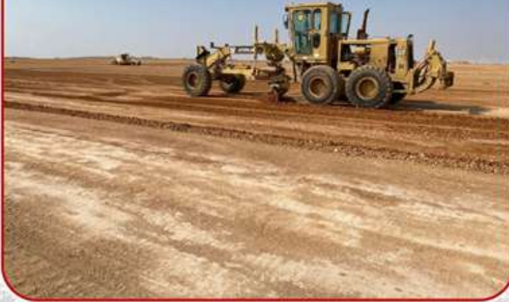
Scope-05 Civil Earth Works
