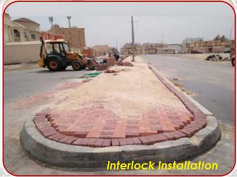
Scope-06 Interlock Installation
