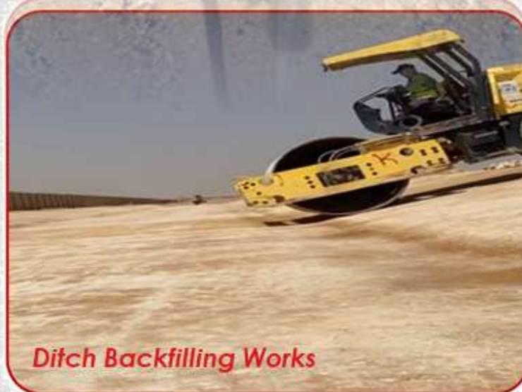
Scope-04 Supply & Apply Backfilling Works
